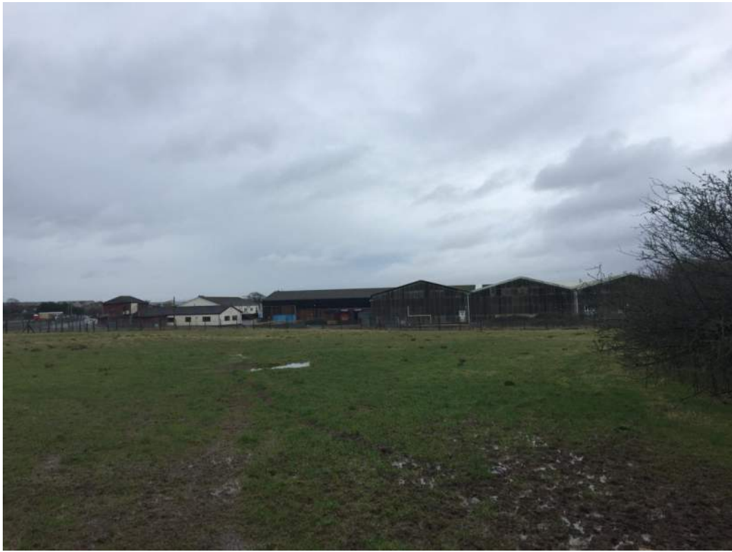
Photo 3: Looking east – warehouses and office buildings of the disused abattoir.
