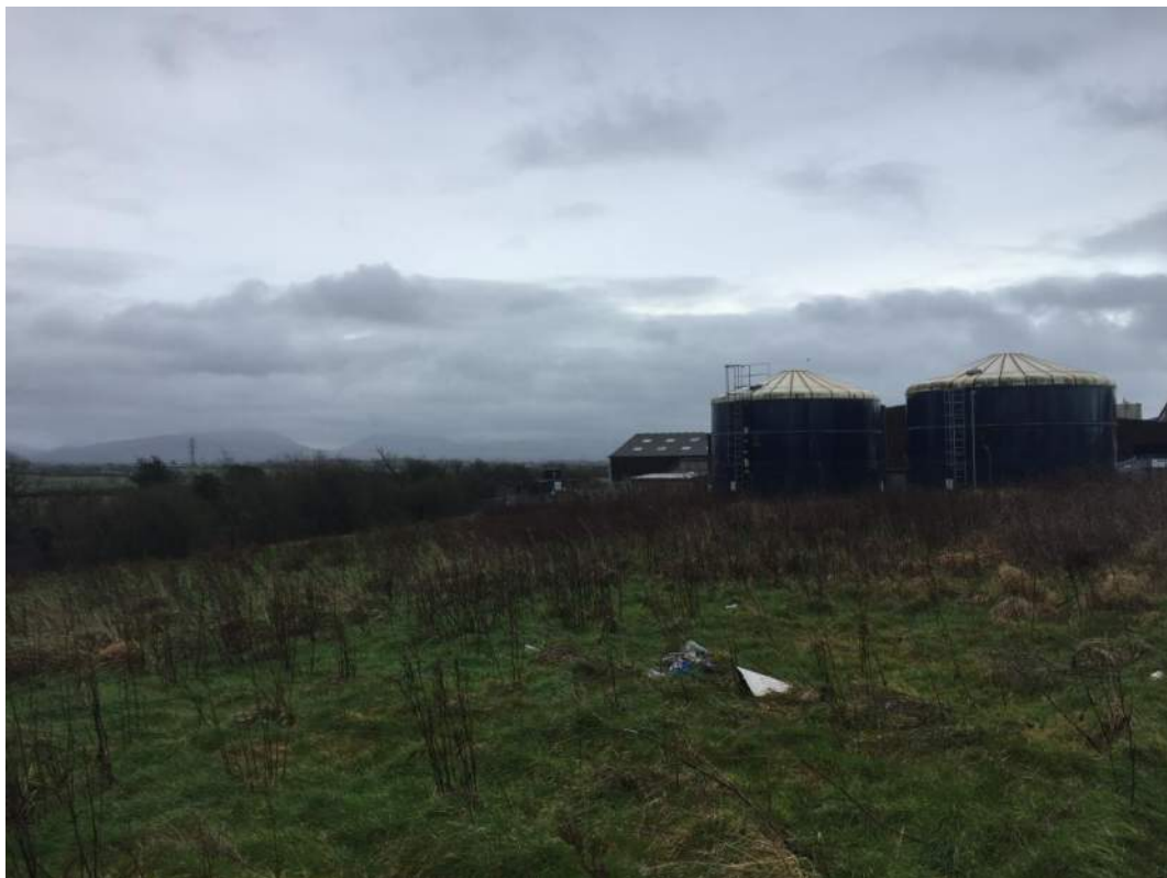
Photo 5: Water storage tanks near the eastern boundary.
